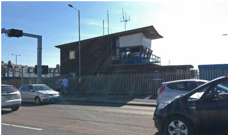
Figure 68: Photograph of existing A47 Bascule Bridge control tower
