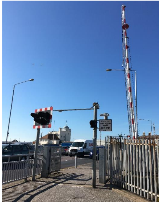
Figure 42: Photograph of wigwag warning lights and barriers on the A47 Bascule Bridge
